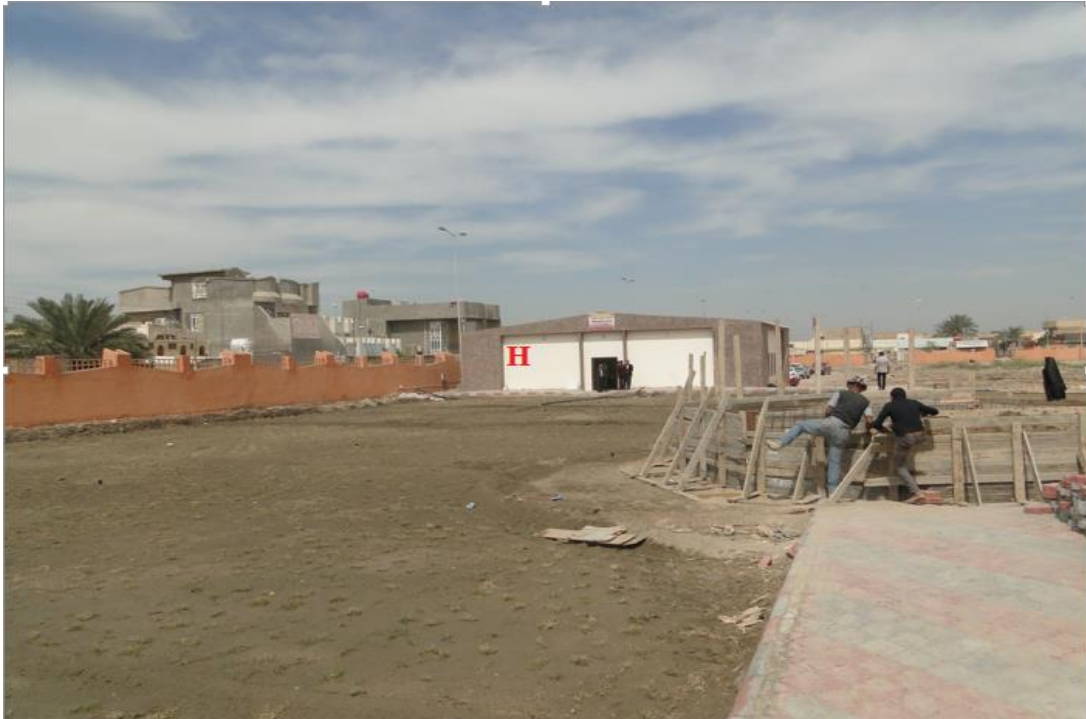
Figure 5-ground picture new buildings are started constructed2014.
