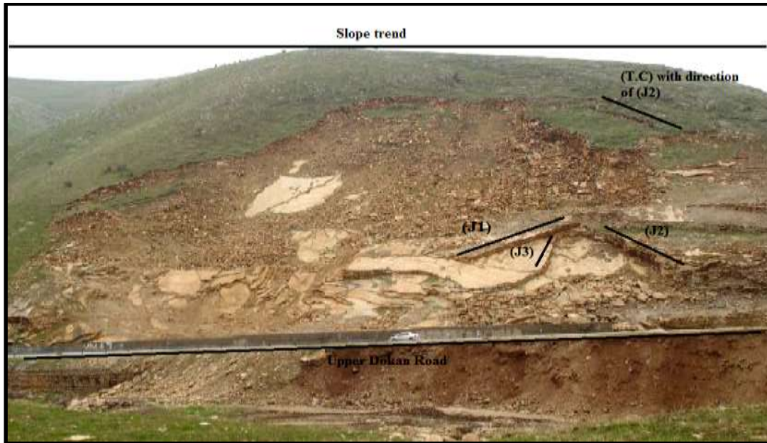
Plate1- General view for station no.1. Photo was taken in the SW-direction.
