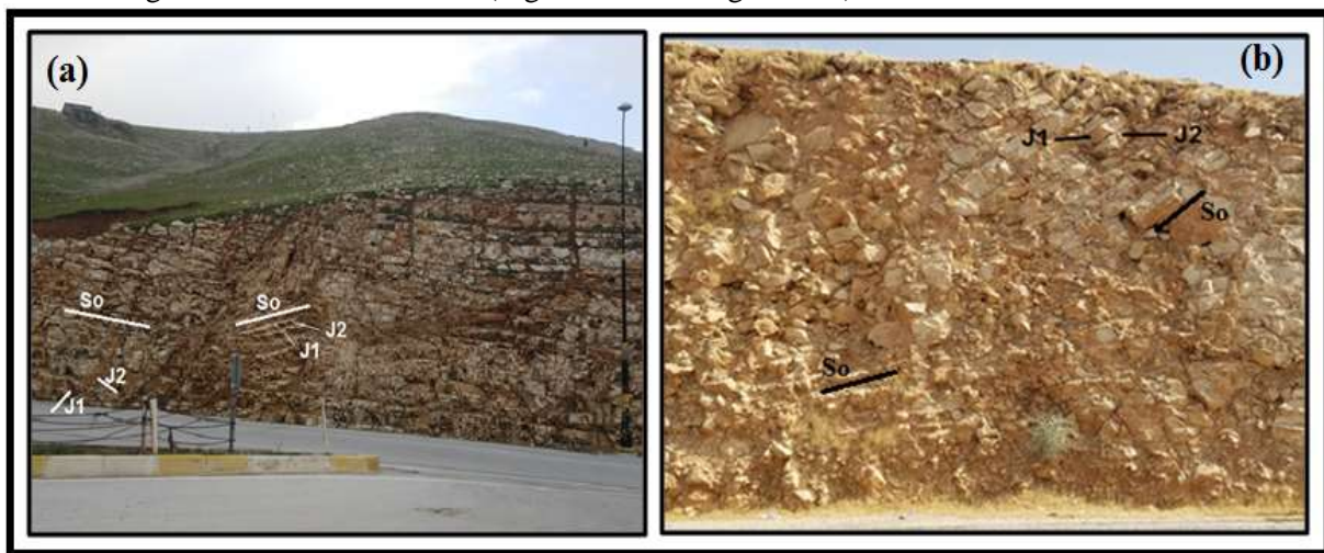
Plate 9- (a) Frontal view showing the slope of left side of station No.9 with Joint sets No.1 (J1) and No.2 (J2) of each limb of the syncline and bedding plane (So). Photo direction is NE. (b) Frontal view showing the slope of right side of station No.9 with Joint sets No.1 (J1), No.2(J2) and bedding plane (So). Photo direction is NE.
