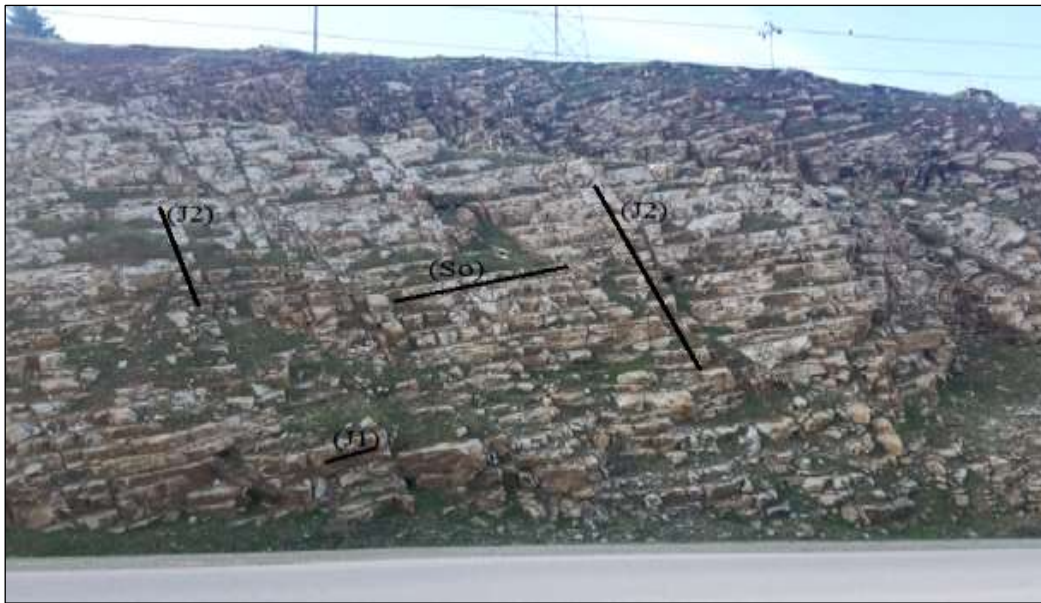
Plate 5 -Frontal view showing the slope of station No.5 with Joint sets No.1(J1), No.2(J2) and bedding planes (So). Photo direction is SW.
