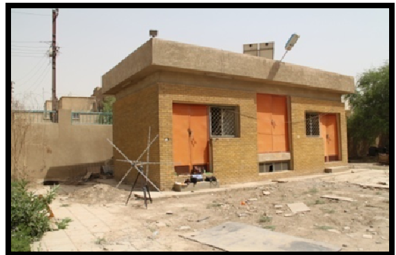
Figure 6- The Photos Of The Building With Control System.
