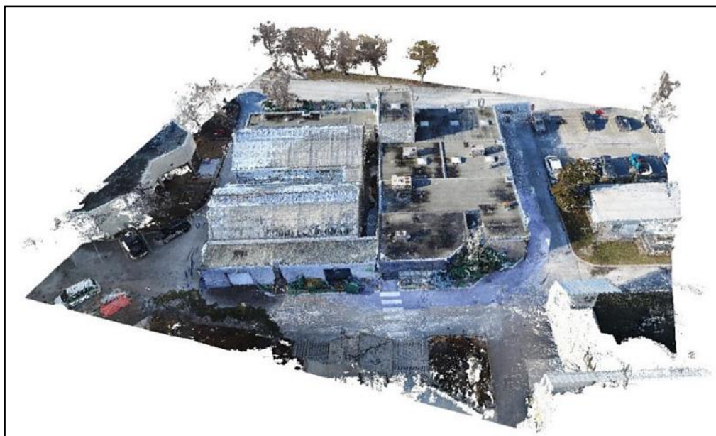
Figure 16: Final 3D building model from fusing photogrammetric/UAS and TLS point clouds [18].
